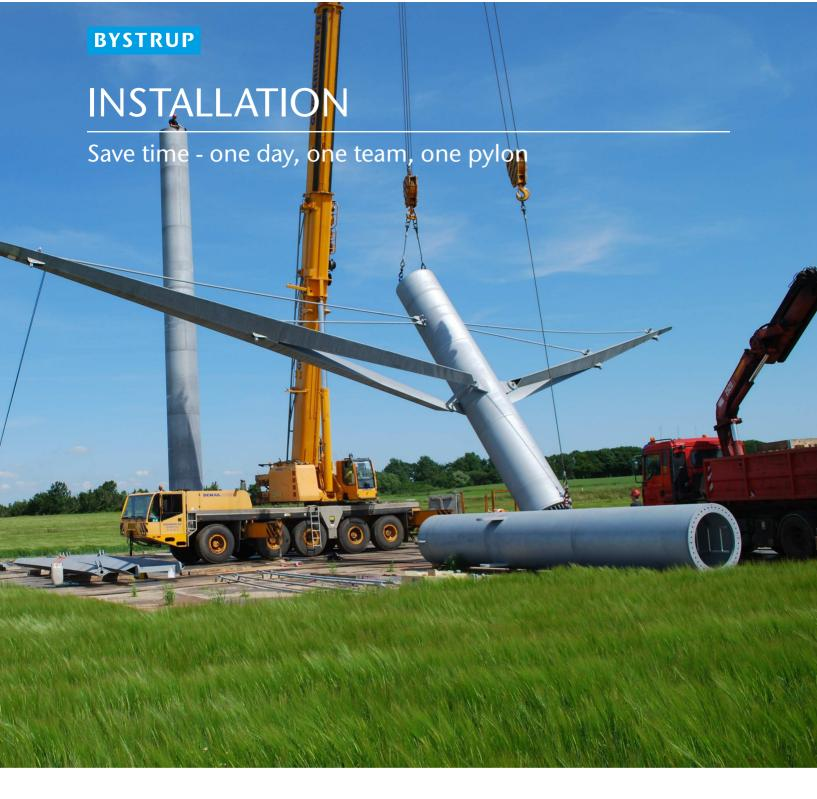
The construction of power pylons has traditionally been a time consuming process. However, with modern manufacturing processes and elements that can travel on the road in a few pieces, it is possible to erect a pylon a day.
