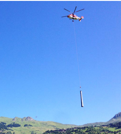
A section of the pylon arrives
